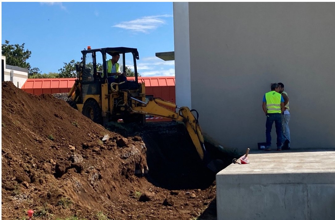
Fig. 13 – Early days of the work for the installation of the building for DRS and AIR Data Center
